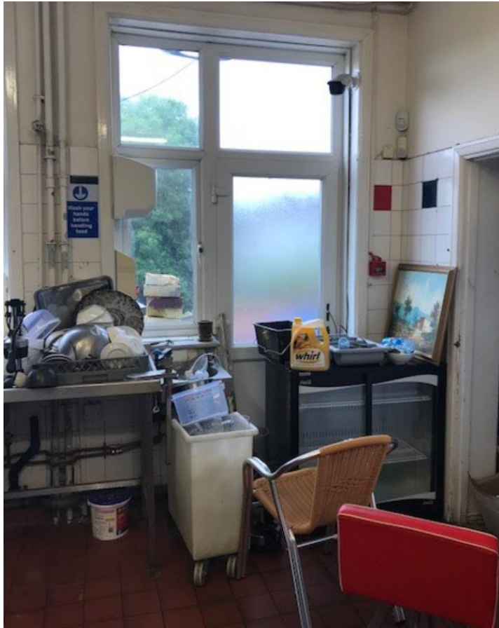
sf057 - Kitchen – Fire exit blocked internally and externally Photograph taken on 13 June 2019 @ 12.47hrs
